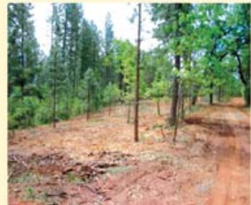
Fuel Break Construction
